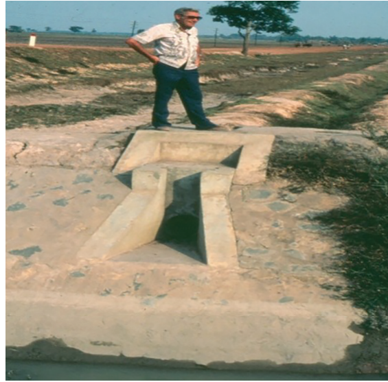
Photo 9.1. Inadequate Design: A Lack of Water Control Structures at Construction, Later Built by Farmers Using Local Materials
