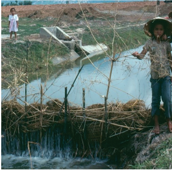
Photo 9.1. Inadequate Design: A Lack of Water Control Structures at Construction, Later Built by Farmers Using Local Materials
