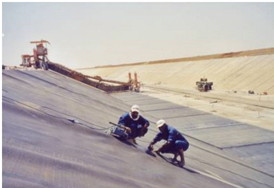
a. Egypt: Toshka Canal HDPE Geomembrane Protected with Fiber Concrete
