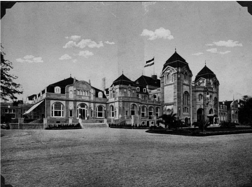
Bad Neuenahr—The Casino
