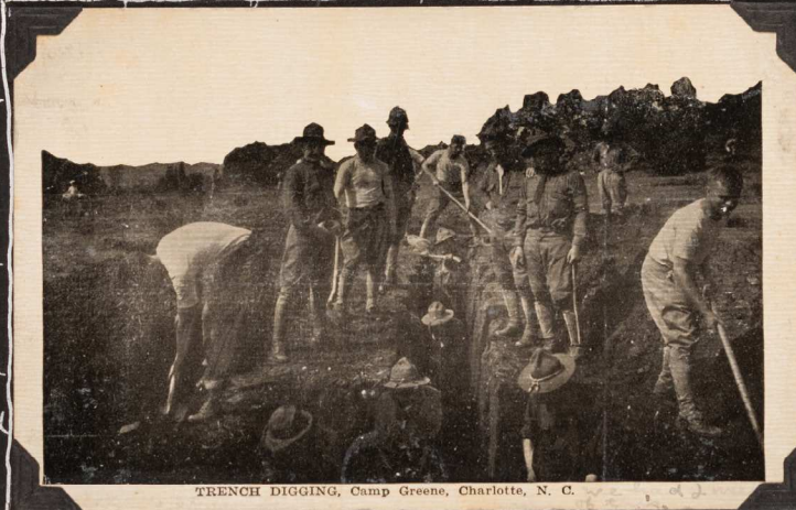
TRENCH DIGGING, Camp Greene, Charlotte, N. C.
