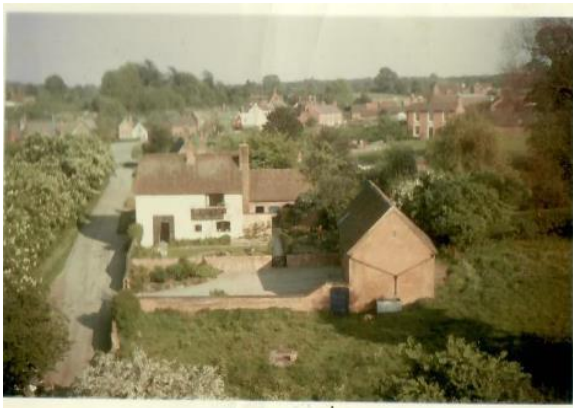
Figure 2: Church House in 1964 - view from the Church Tower
