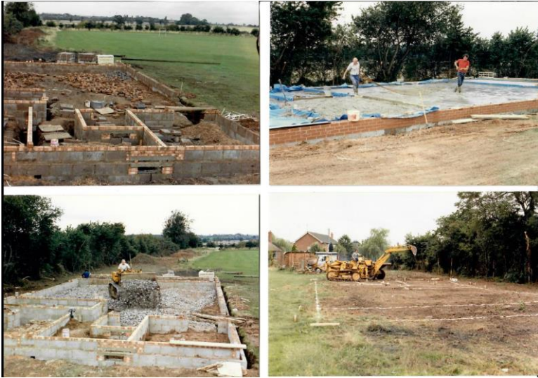
Figure 14: Building Work Stage One - 1986
