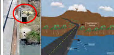
Non-Contact Measurement of Stage & Discharge
